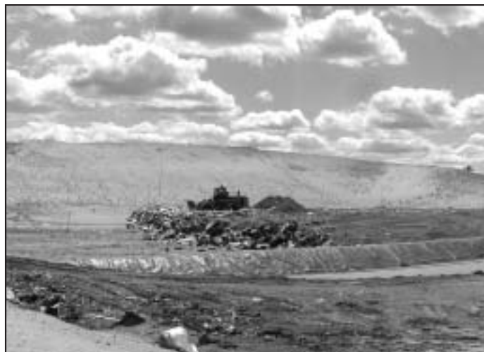
Full-scale bioreactor landfill allows direct evaluation of design and operation.
